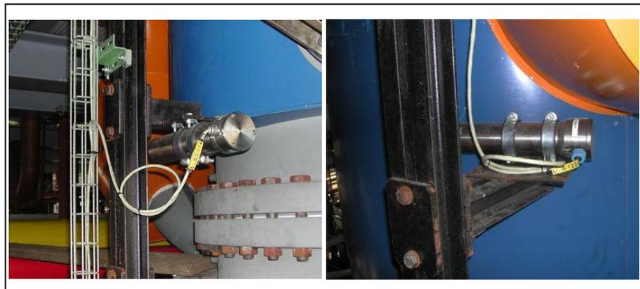
**5.2.4 Installation of the GM Detector**
